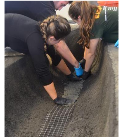
Figure 10: Placement of Spine and Structural Layer
