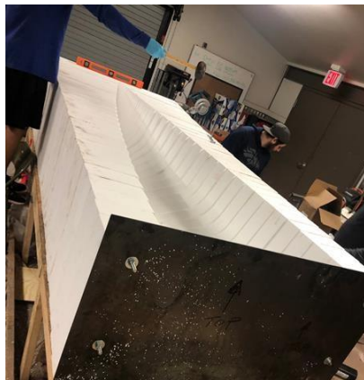
Figure 6: Mold Construction in Progress
